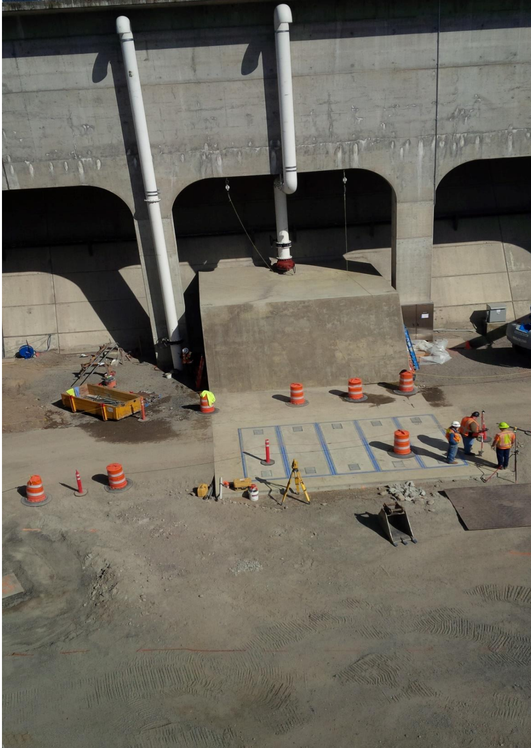
AWS construction completed 10' valve room. Ready for commission testing next week.
